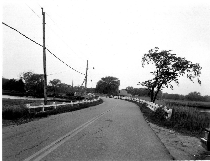
APPROACH (LOOKING WEST)
