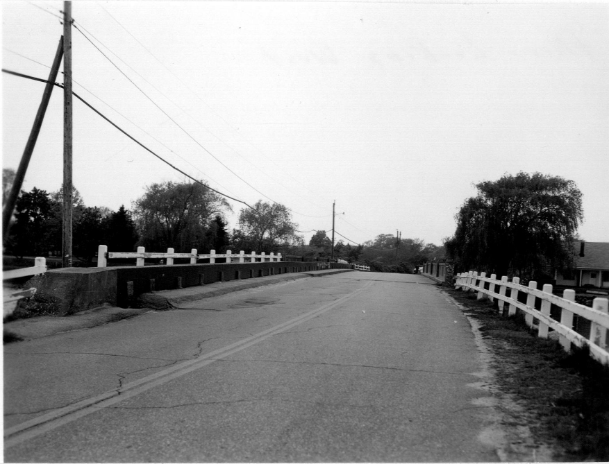
THRU - LOOKING WEST
