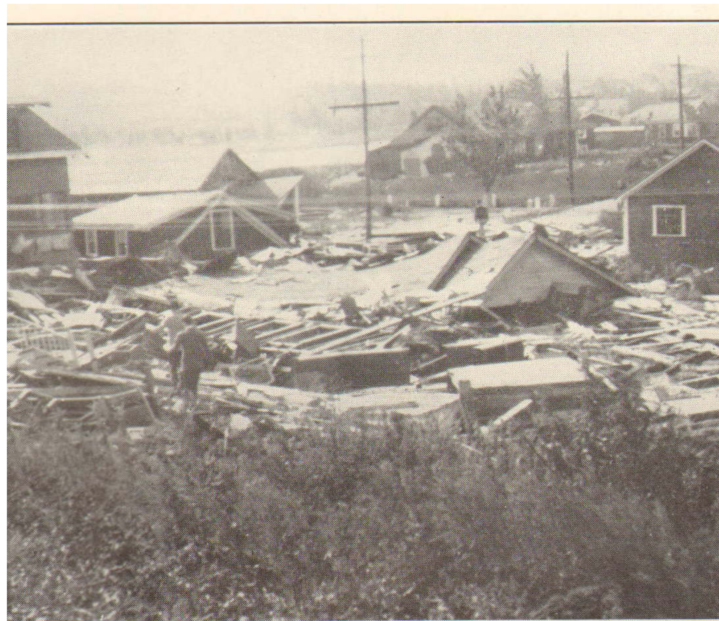
f year-round homes at Ocean Grove which were ripped from foundations
